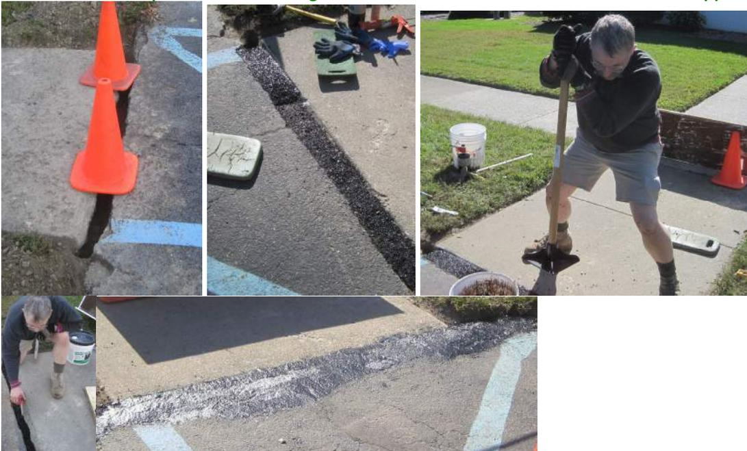
Repair of the Handicap parking Area. A dangerous divot formed, now repaired with crack filler.
